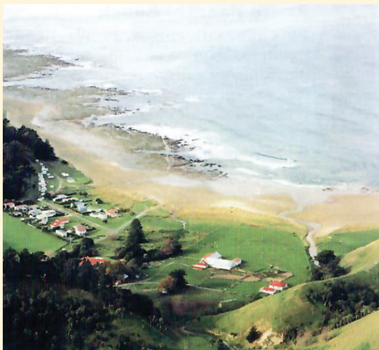
Photo by Survey Services.
