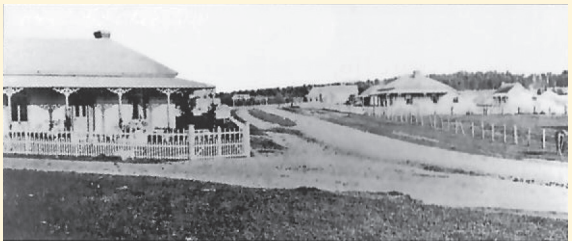
Pre 1880s view looking south along Wellington Road.
